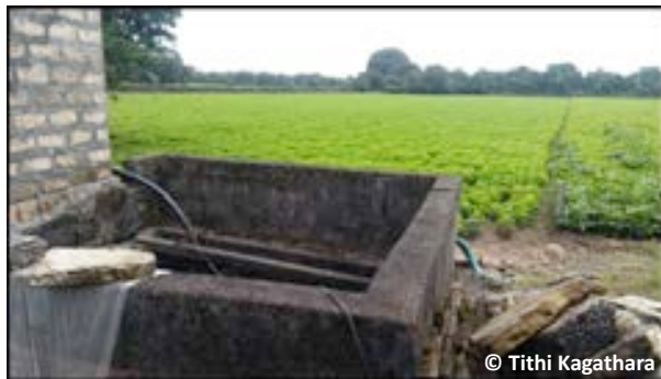
Image 2. A well with the parapet wall.
